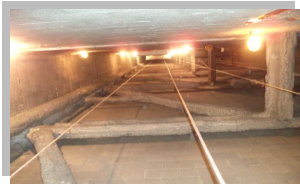
The airshaft at the Maricopa County east court building in 2014.
