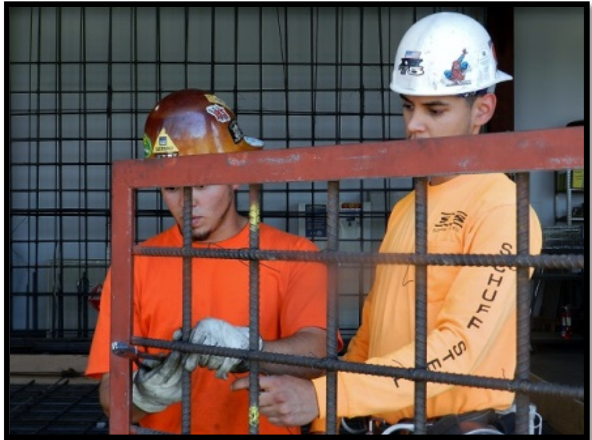
Ironworkers Local 75 apprentices practice cutting wire at the training center.
