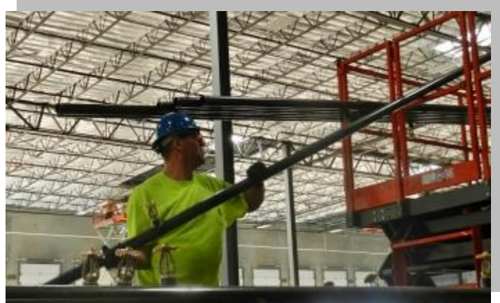
UA Local Union 669 at Marshall's Distribution Center project. Goodyear, Arizona.
